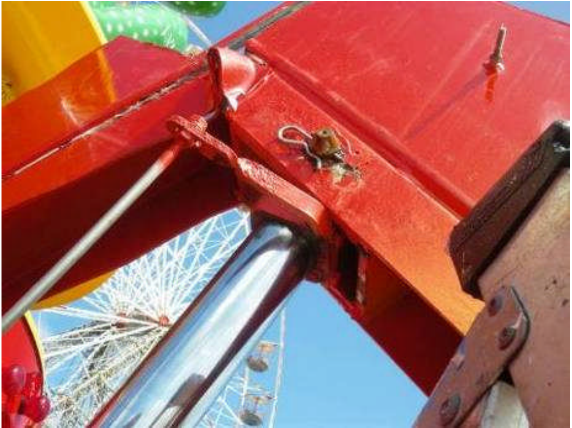
IMGP1566 – Lower Stiffer and Lift Point Strengthening Plates
