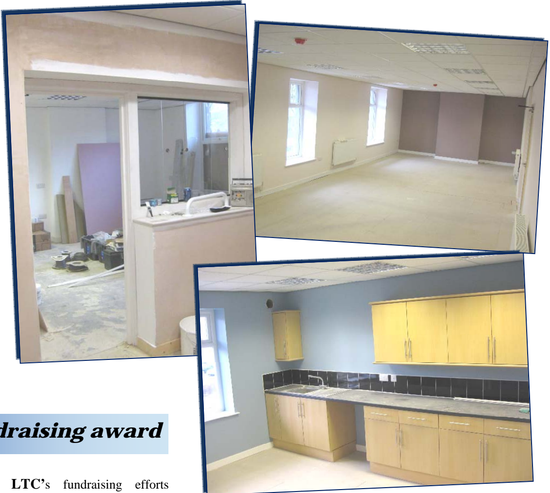
Above: Views of the new office space during refurbishment
